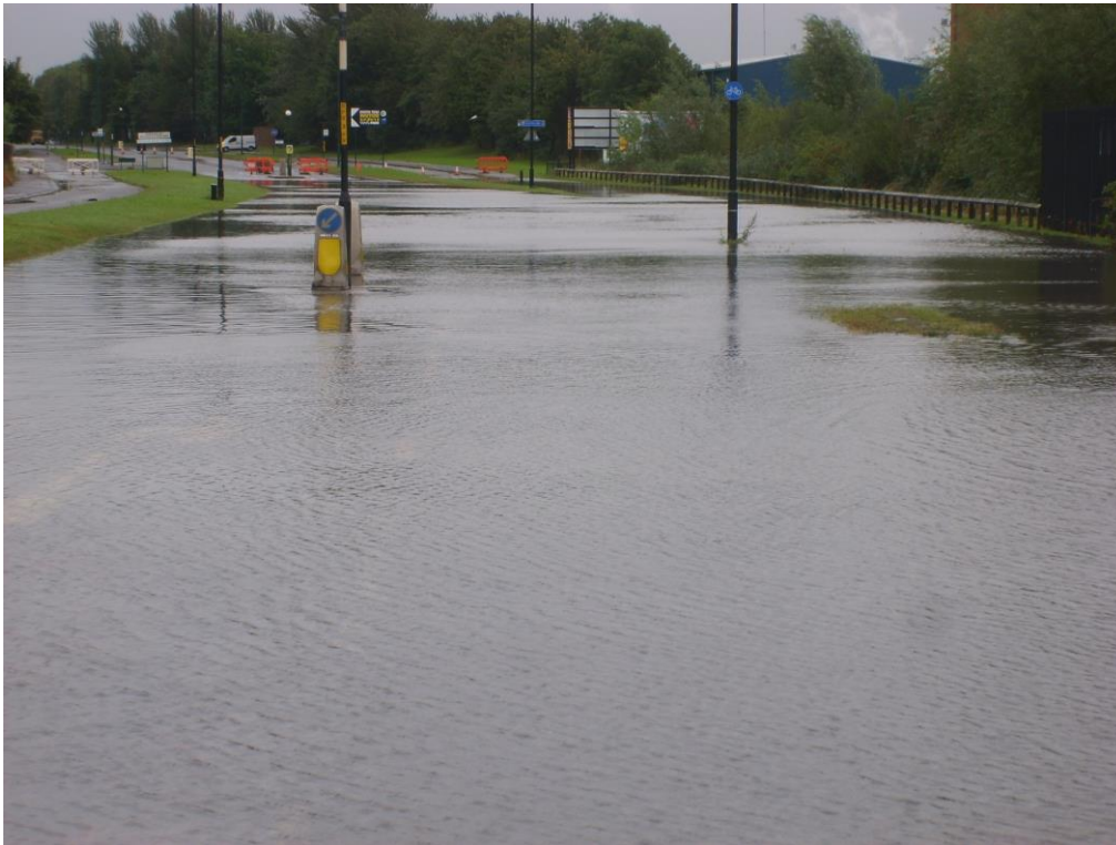
Figure 7 Flooded South Bank Road
