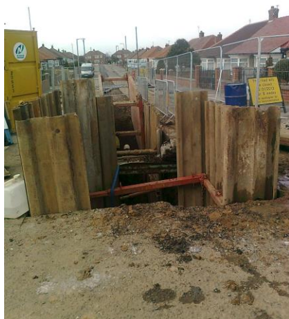
Figure 11 Holbeck Avenue works
